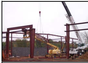
Coleman Suzuki Construction Site
