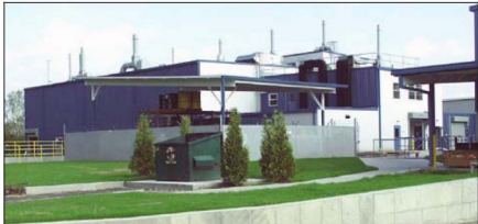
Completed in 2002, the construction of a combined office-warehouse building and specialty manufacturing facility marked the beginning of our relationship with Gelest, Inc. The new facility allowed Gelest to transition from a start-up to a true mid-sized manufacturing company.
