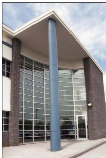
The office's exterior combines EIFS, rock faced masonry units and aluminum composite panels with generous fenestration.
