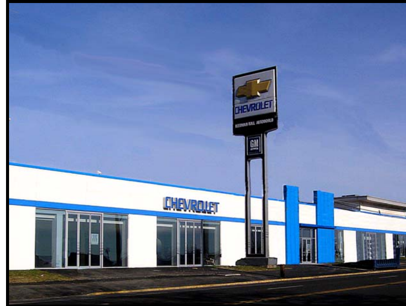
New window and door openings are set into an EIFS background. Preformed blue metal panels were used to create the entry tower for the Chevrolet showroom.
