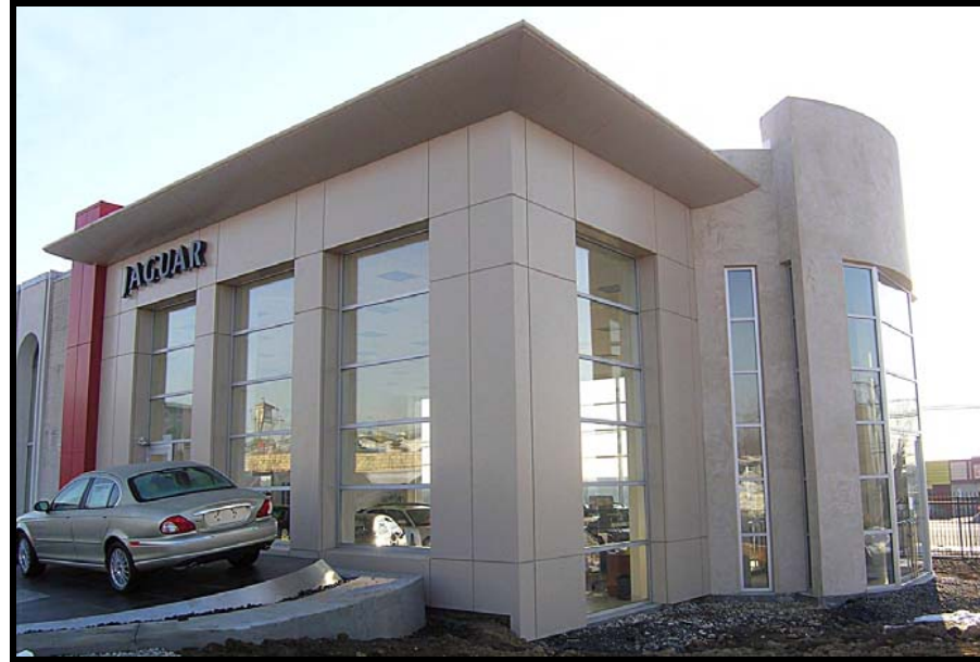
Aluminum wall and curved canopy panels set the Jaguar showroom apart from all other brands. A two story stucco entry tower caps the south end of the “running quarter mile”. (Rear)
