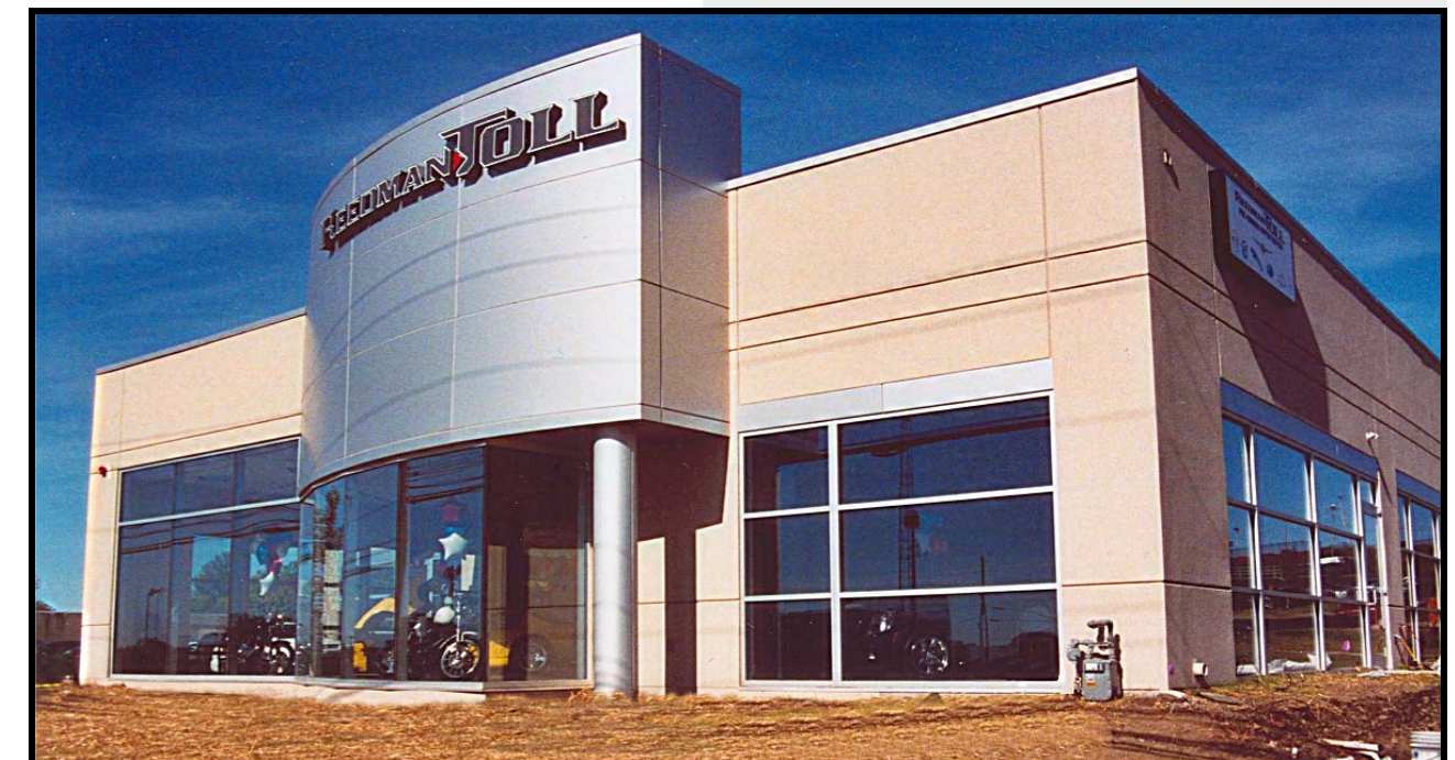
The original 2,250 SF car appraisal building now measures 6,633 SF and has become the Pre-owned Supercenter. The exterior includes composite metal panels, EIFS and a circular storefront glass system capturing both north and southbound traffic along Business Route 1.
