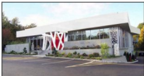
EFS and poured concrete exterior finishes are offset by a distinctive portal designed to have the look of a Cortain finish.
