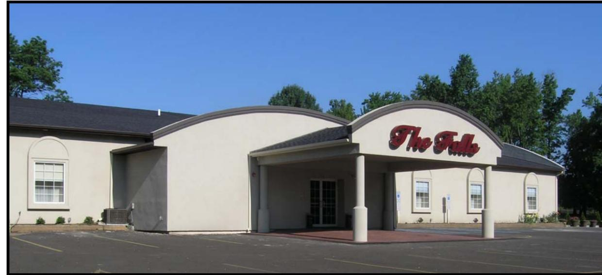
The entire exterior theme was reset from multiple "A" roofs to softer rounded parapets and end walls. All horizontal wall surfaces received EFIS (a lightweight stucco system) which really brought out the fan topped window detail. A new entry canopy and stamped concrete floor provide safe and comfortable entry and exit to and from The Falls.
