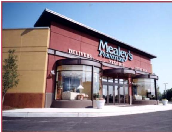
Using innovative materials and construction techniques to accomplish the planned effect, Penn Valley Constructors began its work at the Fairless store by adding 31,800 square feet to the existing building. A new curved glass front entrance facade was further enhanced by two elevations of rich and colorful EIFS.
