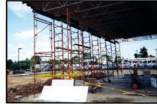
Temporary wall bracing
