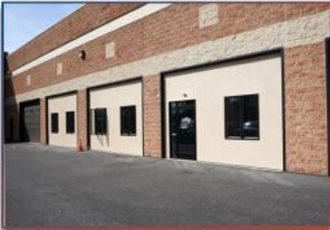
Three overhead doors were replaced with EIFS, new doors and windows. A portion of the warehouse was converted to an open floor plan office with new bathrooms, break room, training and conference rooms.
