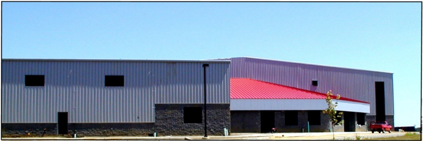
Right wing houses soccer arena and roller rink at 192' x 90' each. Left wing for future Gold's Gym at 22,000 SF. Note: Progress photo, three months prior to completion.
