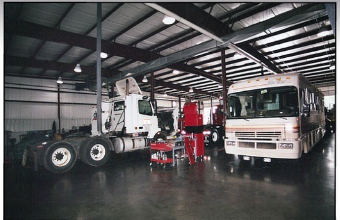
The overhead carbonic exhaust system includes eight exhaust stations positioned throughout the truck shop.
