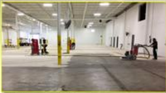
Grinding down concrete
