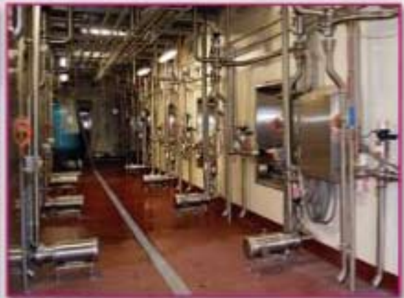
Silo Tank Hall
