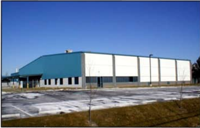
Gelest's Office-Warehouse is a pre-engineered building featuring Dryvit, metal siding, rockface and painted block. Vapor detection and emergency ventilation are included to meet the requirements of NFPA 69.
