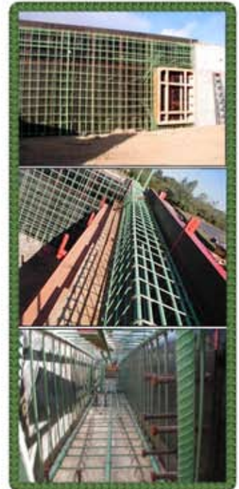
Reinforcing steel bars with an epoxy coating are used to provide "DLC".
