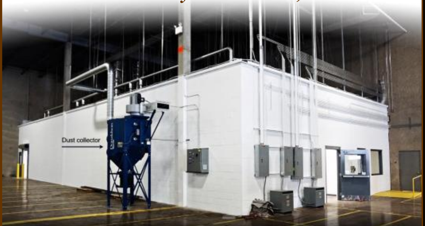
Outgoing preparation room exterior with dust collector
