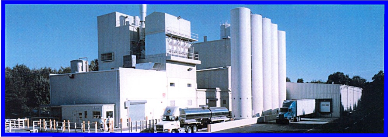
Dryer #4 with baghouse, transfer station and bulk 50,000 gallon tanks
